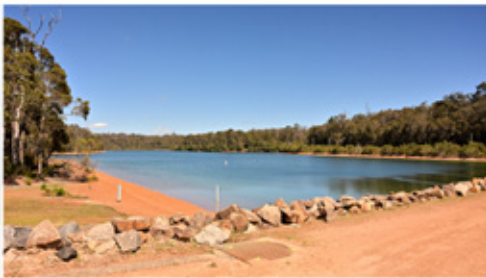
Ten Mile Brook Dam
